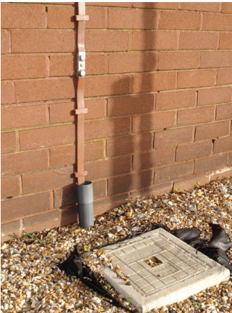
Figure 51. Typical down-conductor connectors.
