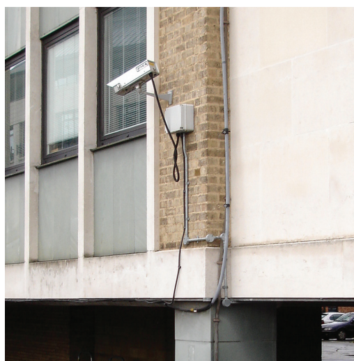
Figure 65. Conventional down-conductor separation distance problem.
